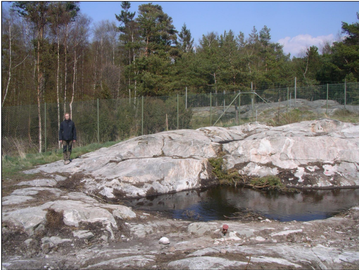
Puddle before being drained by channeling, location coincident with northern wall of the building. The cored borehole (red metal cover) is visible in the foreground.
