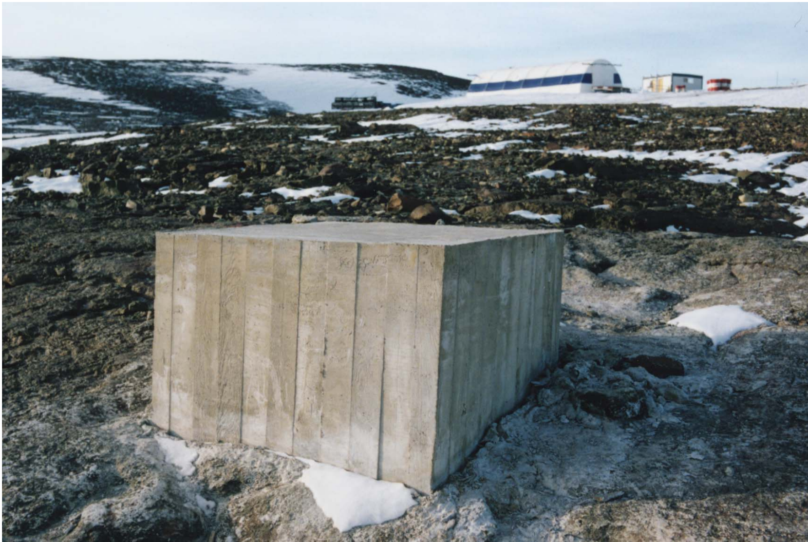
Aboa absolute pier 0.56 cubic meters, density 2.2 \times 10^3 \text{ kg m}^{-3} , mass 1.2 \times 10^3 \text{ kg}
